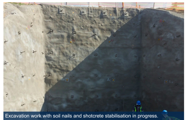
Excavation work with soil nails and shotcrete stabilisation in progress.
