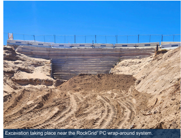
Excavation taking place near the RockGrid® PC wrap-around system.
