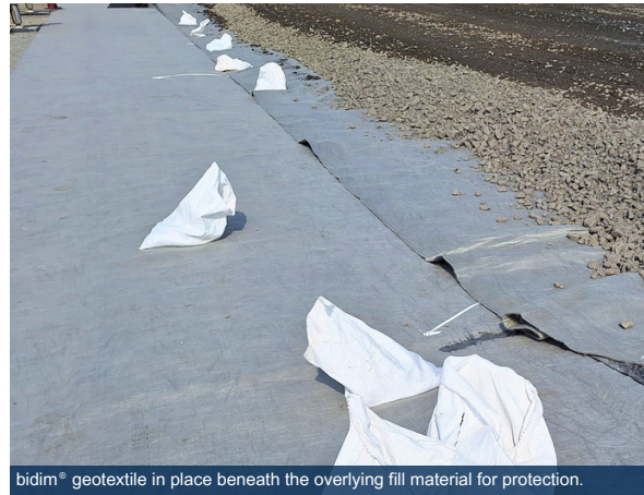
bidim® geotextile in place beneath the overlying fill material for protection.
