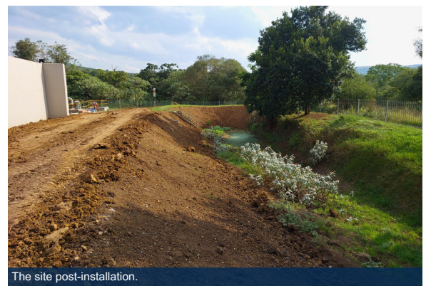
The site post-installation.
