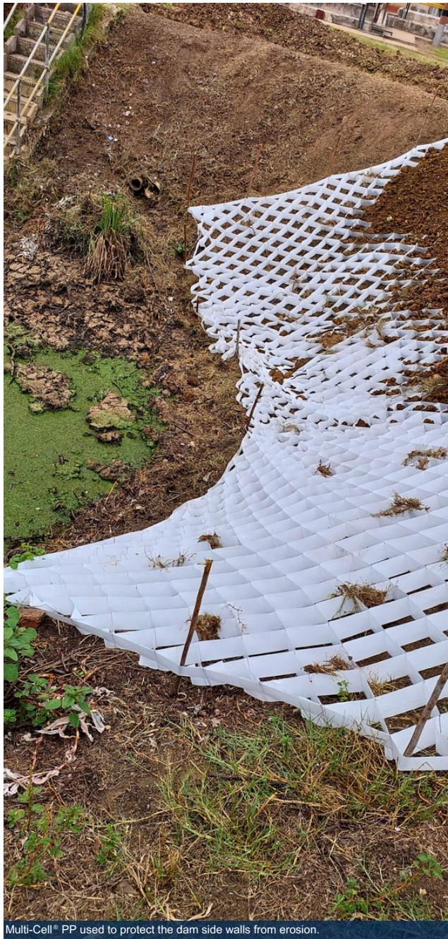
Multi-Cell® PP used to protect the dam side walls from erosion.
