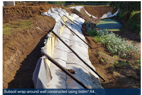
Subsoil wrap-around wall constructed using bidim® A4.
