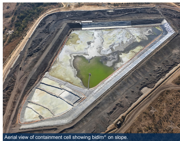
Aerial view of containment cell showing bidim® on slope.
