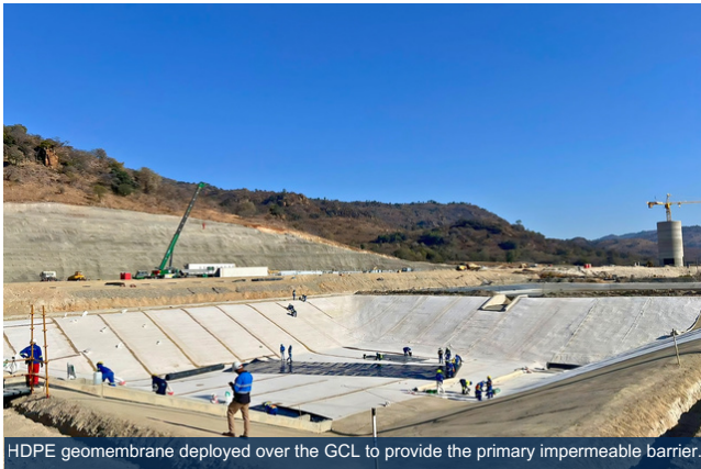
HDPE geomembrane deployed over the GCL to provide the primary impermeable barrier.
