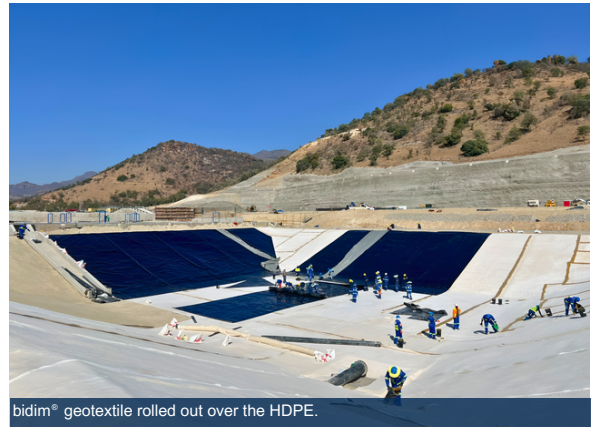
bidim® geotextile rolled out over the HDPE.
