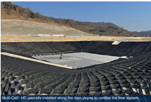
Multi-Cell® HD geocells installed along the dam slopes to confine the liner system.
