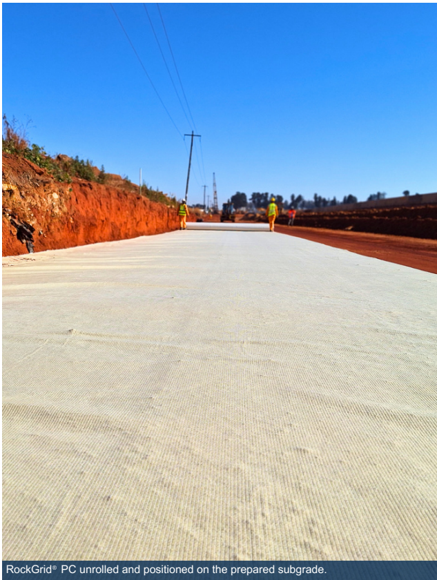
RockGrid® PC unrolled and positioned on the prepared subgrade.
