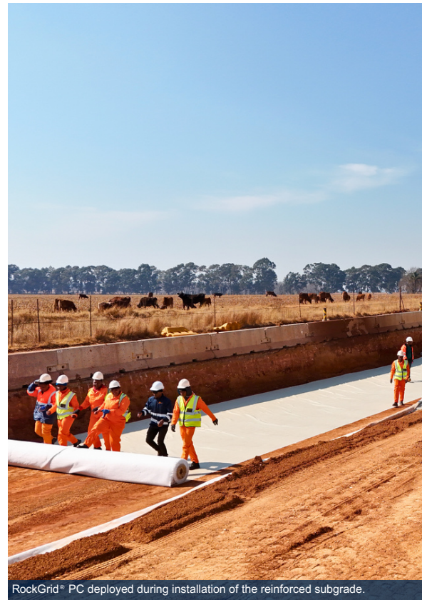
RockGrid® PC deployed during installation of the reinforced subgrade.
