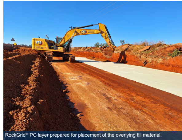
RockGrid® PC layer prepared for placement of the overlying fill material.
