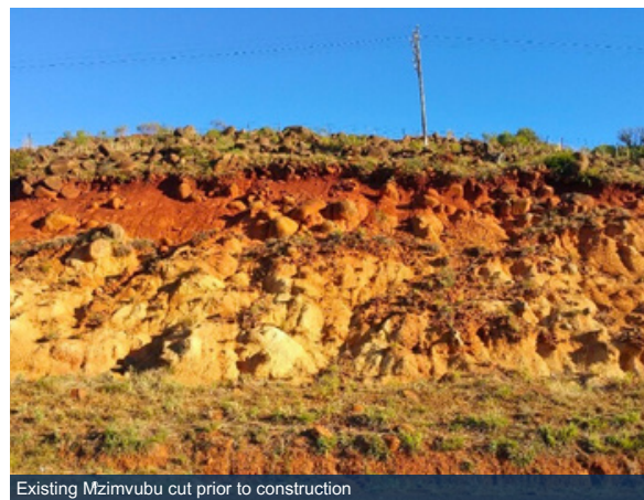
Existing Mzimvubu cut prior to construction
