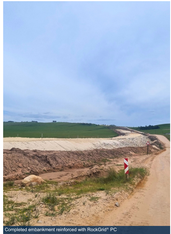
Completed embankment reinforced with RockGrid® PC
