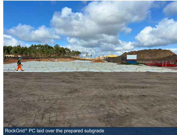
RockGrid® PC laid over the prepared subgrade
