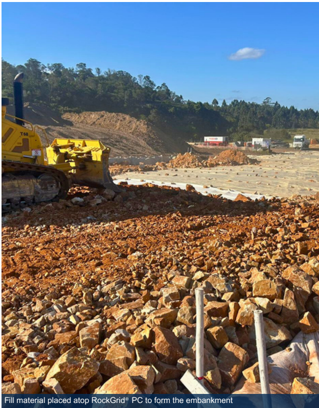
Fill material placed atop RockGrid® PC to form the embankment
