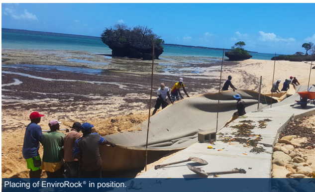
Placing of EnviroRock® in position.
