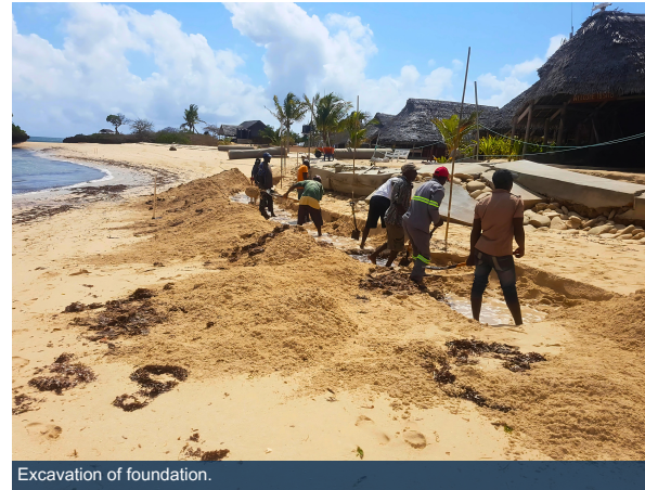
Excavation of foundation.
