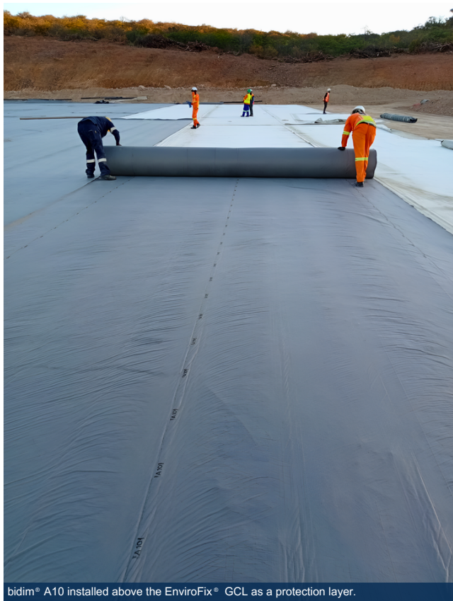
Protected liner system forming a stable working platform during construction.
