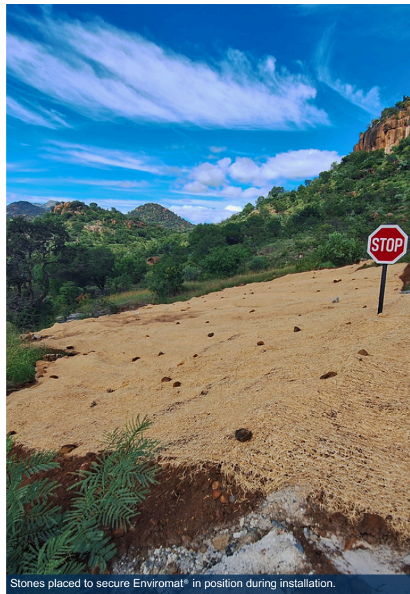
Close-up of Enviromat® installed on haul road side slope.
