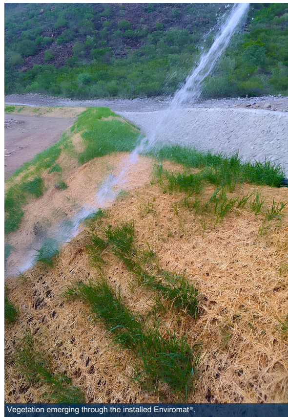
Vegetation emerging through the installed Enviromat®.
