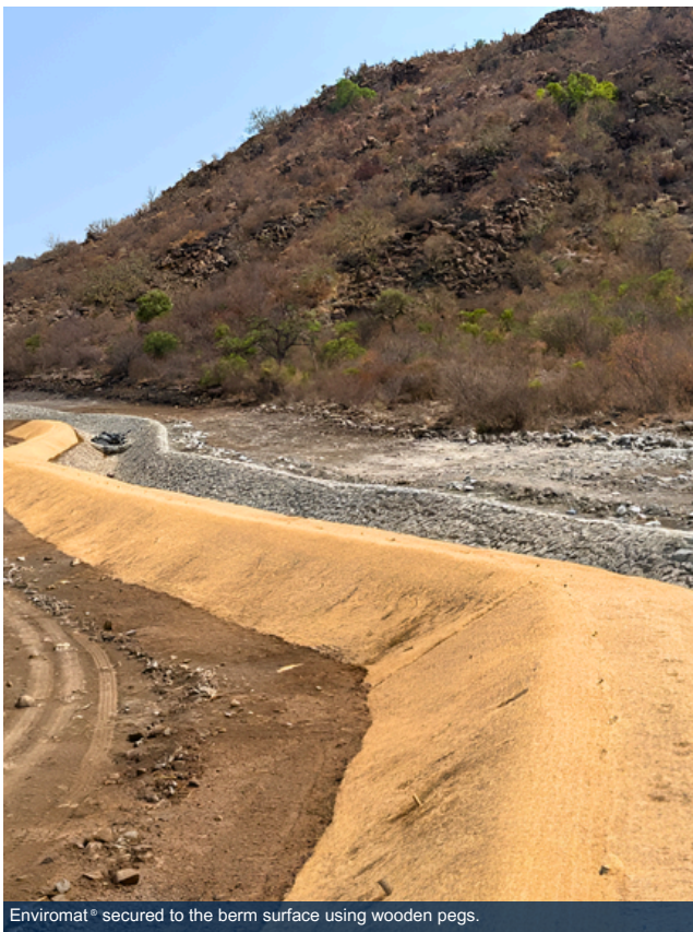
Enviromat® secured to the berm surface using wooden pegs.
